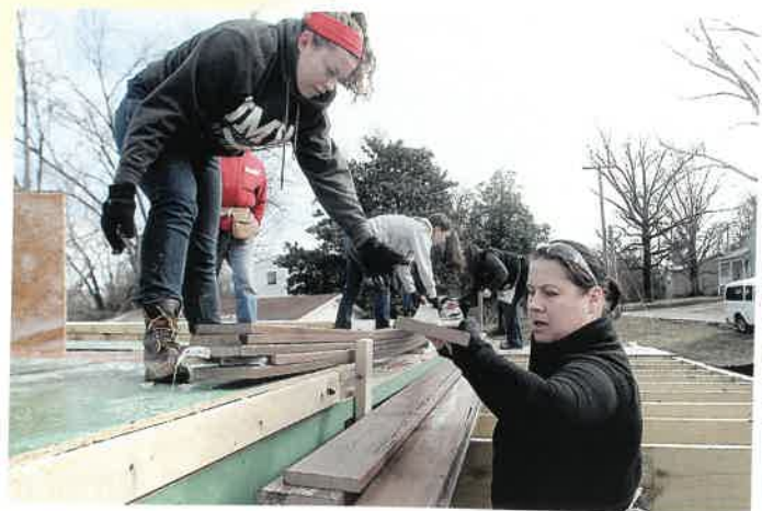
Rachel Sturgis (left) and Dawn White move porch flooring down to the porch at the 2017 Habitat for Humanity Women Build.
